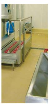
The very chemical resistant nature of UCRETE® industrial flooring means that no commercially available cleaning compounds will damage the floor when used at their normal concentrations. Puddling of cleaning solutions if allowed to evaporate to dryness may lead to deposits on the surface and 'water marks' which can be hard to remove subsequently. It follows that removal of cleaning solutions and adequate rinsing is required to maintain your floor looking its best.
