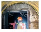
**CROSS-PASSAGE JUNCTIONS** Waterproofing of junctions with connecting galleries and escape routes and/or joining these to main tunnel.
