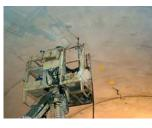
VOID FILLING Injection to fill and seal dry voids and water pockets behind tunnel lining.
